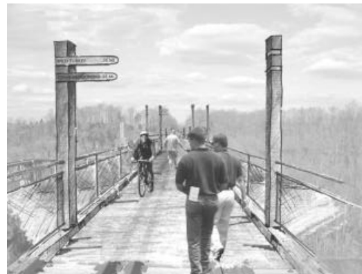
View of proposed rail trail conversion of Young's High Bridge.
